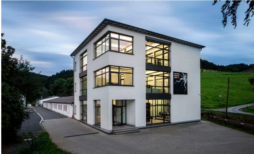
The SON-building for development, distribution and administration.
