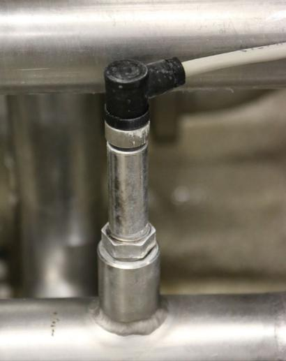
The conductivity sensor CPS-7 makes it possible to detect product changes and determine phase separations in the food and pharma industries.
